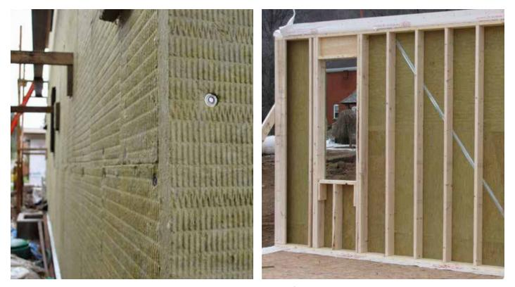
As an exterior insulation, ROXUL COMFORTBOARD 80 is fastened to the exterior OSB/plywood sheathing or structural stud wall and is designed to provide increased thermal performance to the building envelope
