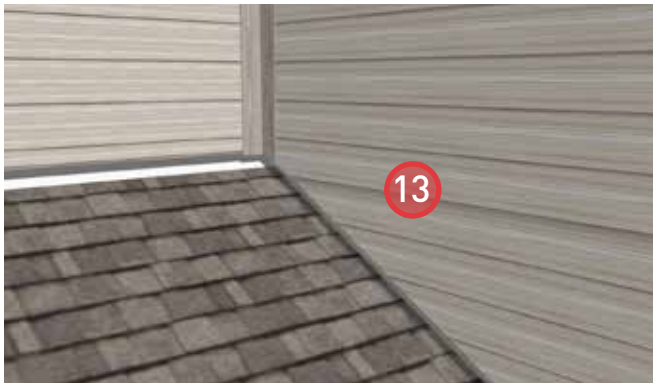
13. Install cladding and trim.
