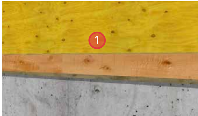
1. Typical wood frame construction at sheathing installation stage.
