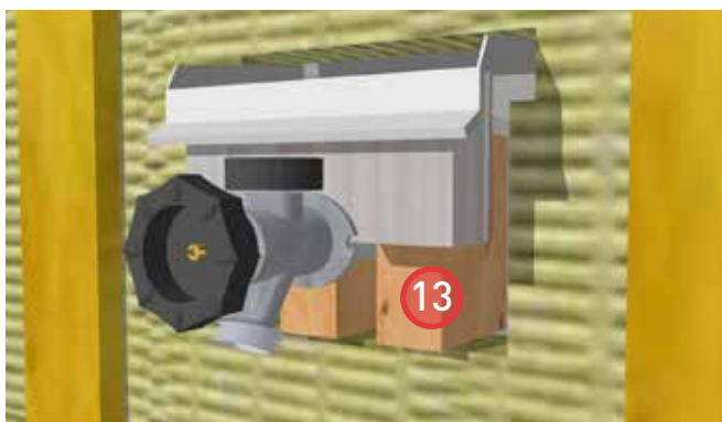
13. Install the top piece of the wood face plate and secure in place.
