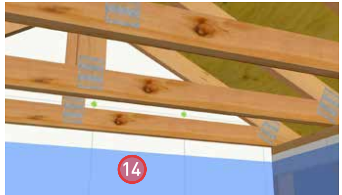
14. Install poly on the walls and fasten to the sheathing membrane with staples.
