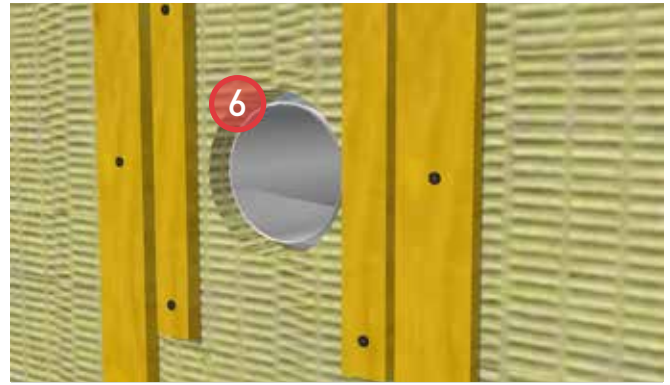
6. Install ROXUL® COMFORTBOARD™ 80 and strapping. Provide bugscreens at the top and bottom of the strapping. Provide strapping around penetration to support the adaptor flange.
