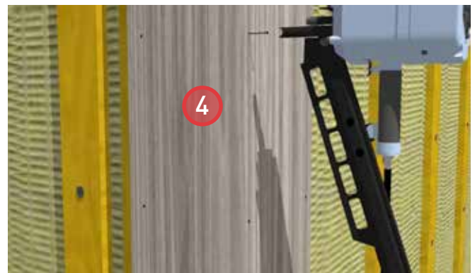
4. The corner trim boards must be nailed together as well as to the strapping to form the corner.
