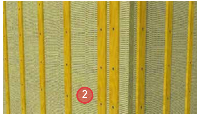
2. Install ROXUL® COMFORTBOARD™ 80. Use the strapping to support the insulation and secure in place with recommended fasteners. Provide bugscreens at the top and bottom of the strapping.
