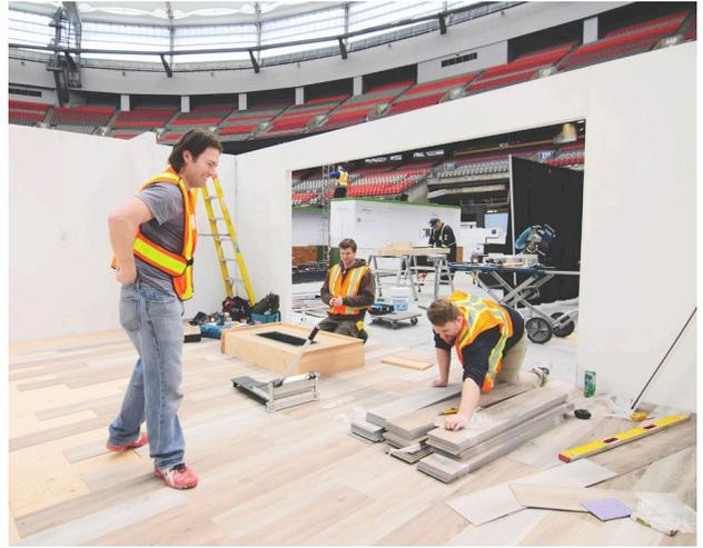
trowel apply an 8" (20cm) wide band of pressure-sensitive adhesive around the perimeter of the room. We recommend Mapei Eco 350 or Taylor 2037. Make sure you let the adhesive dry completely. You should be able to put your hand on the glued area and get no transfer on your hand before starting. Then lay the planks or tiles nice and tight together.
